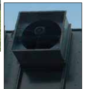
Close-up of Aagaard sound insulated reverse-air fan.
