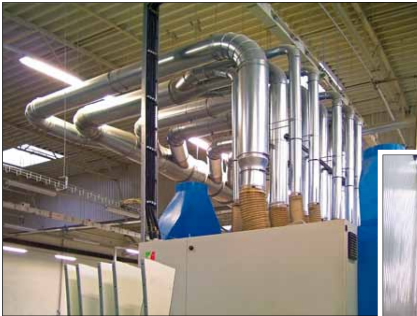
Aagaard chain filter at Danish pinewood furniture factory - air volume: 120,000 m 3 /h.
