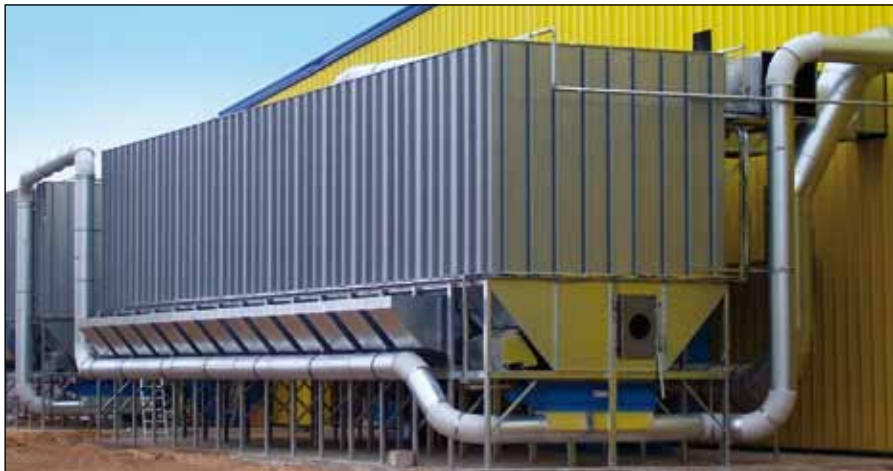
Aagaard chain filter with hopper-mounted explosion relief doors at a factory in Belarus – air volume 250,000 m³/h.
