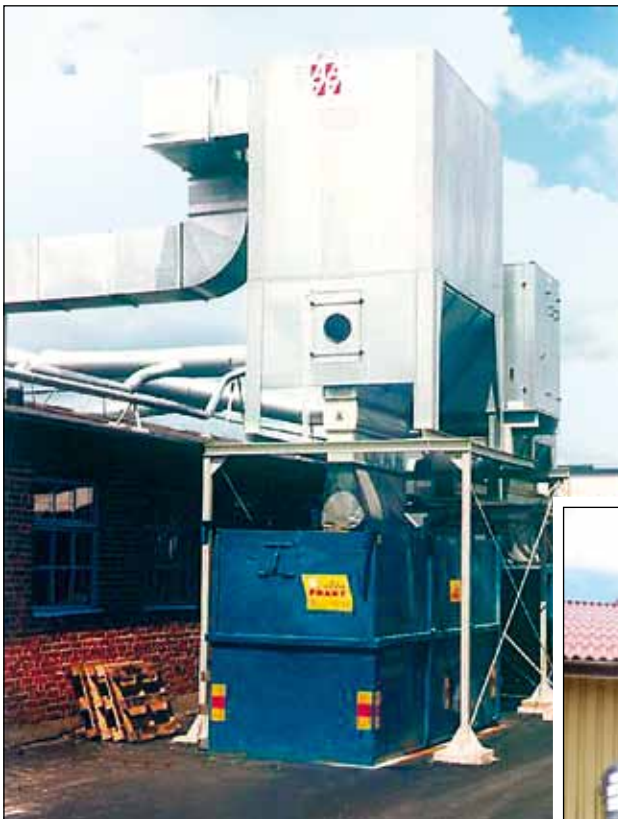
Agaard rotary valve filters on standard Agaard container stands.
