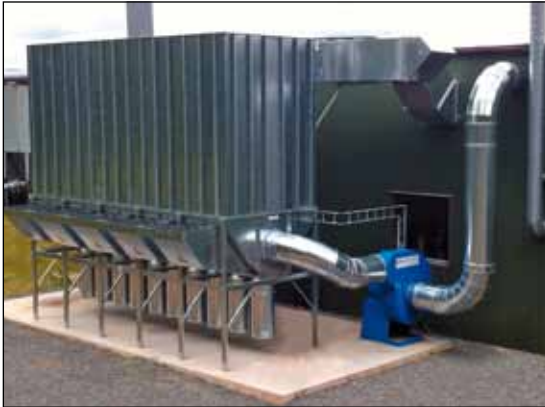
Agaard bag-emptying filter with hopper-mounted explosion relief doors (ATEX approved) and steel bins at Swedish kitchen manufacturer – air volume 45,000 m³/h.
